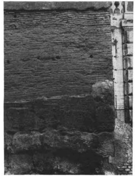
Fig. 96c. S. Martino ai Monti, Ninth century basilica, foundation and rising wall of northeast corner of aisle, near apse
